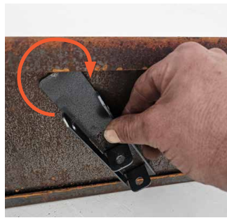
Place the bracket against the back of the edge piece and rotate.
